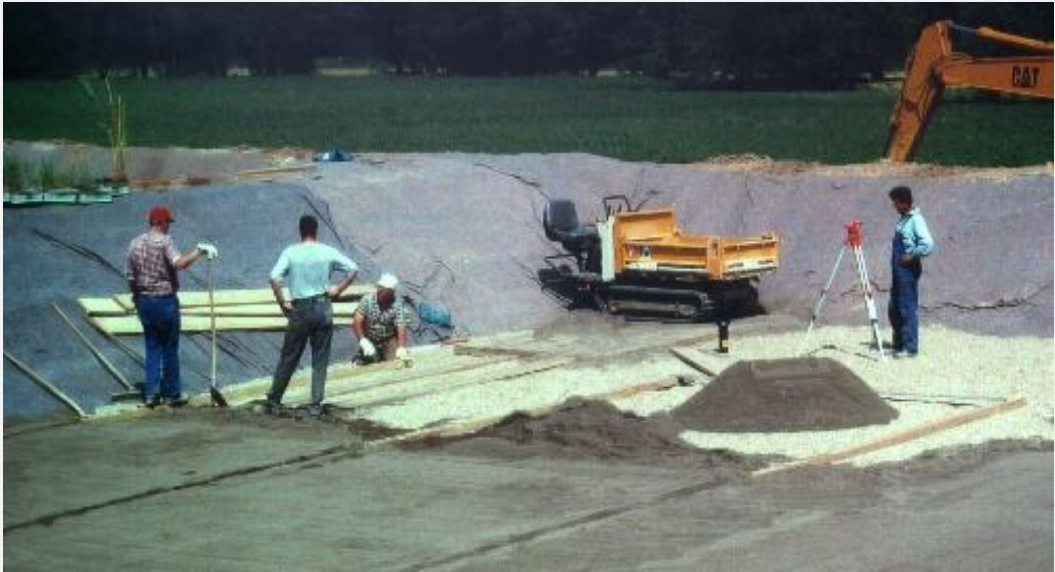
LEVELLING OF THE EXCAVATED REED BED AND LAYING OF GRAVEL AND SAND LAYERS PRIOR TO PLANTING OF REEDS.
